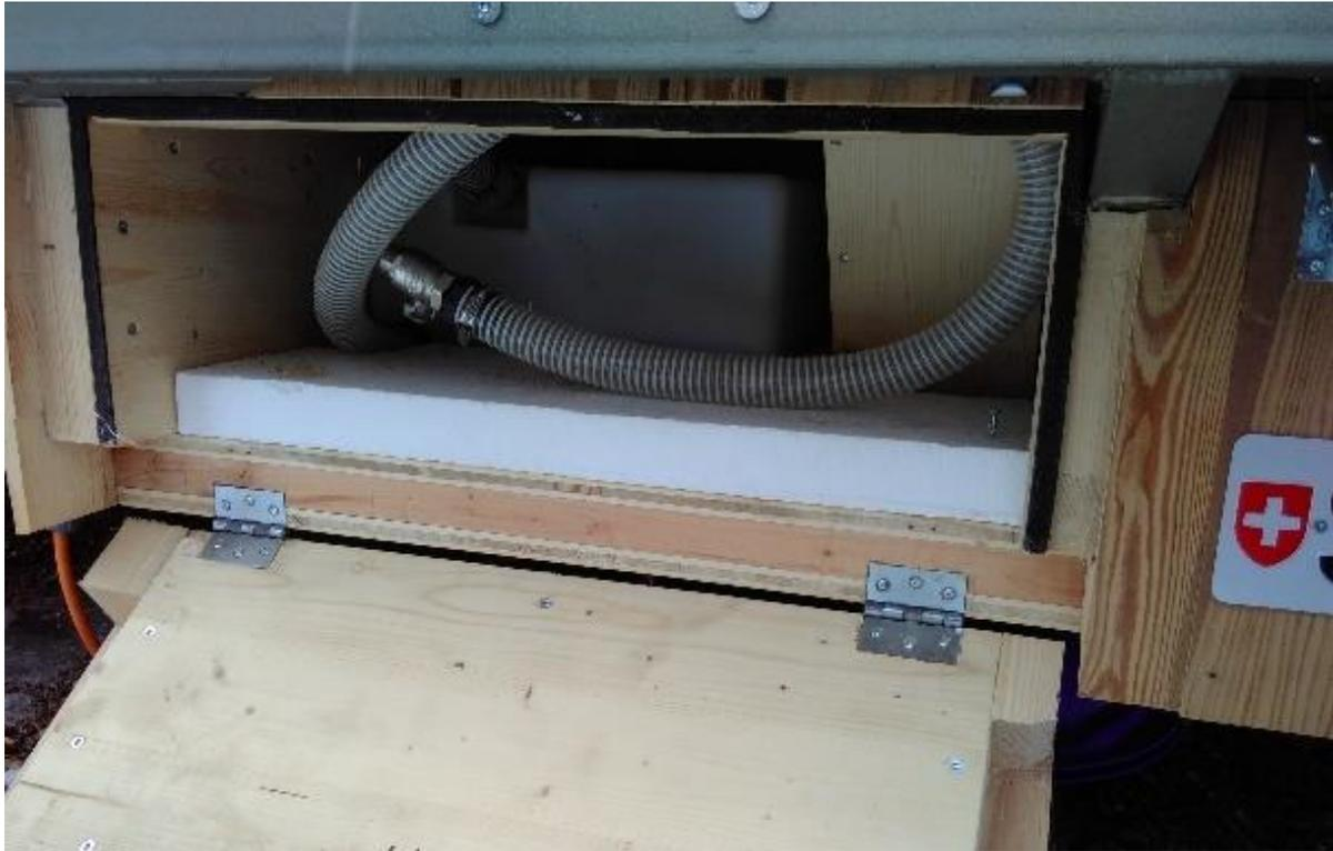
Example of a tank used to store fresh- and greywater
